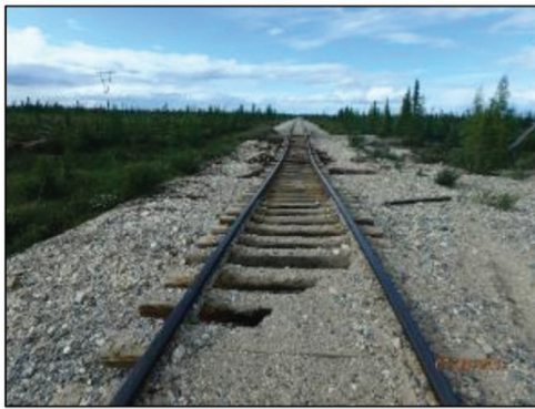
Photos from summer 2017 provided by Omnitrax show washout damage to the Hudson Bay Railway tracks to Churchill. This location was only one of many damaged by the floods that year. Omnitrax chose not to repair the line due to costs, eventually selling it to Arctic Gateway Group. The line has since been repaired and rail traffic has resumed.
