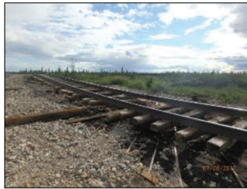
Photos from summer 2017 provided by Omnitrax show washout damage to the Hudson Bay Railway tracks to Churchill. This location was only one of many damaged by the floods that year. Omnitrax chose not to repair the line due to costs, eventually selling it to Arctic Gateway Group. The line has since been repaired and rail traffic has resumed.
