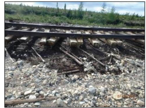
Photos from summer 2017 provided by Omnitrax show washout damage to the Hudson Bay Railway tracks to Churchill. This location was only one of many damaged by the floods that year. Omnitrax chose not to repair the line due to costs, eventually selling it to Arctic Gateway Group. The line has since been repaired and rail traffic has resumed.
